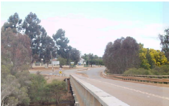
Plate 14: Existing northern entry environment
