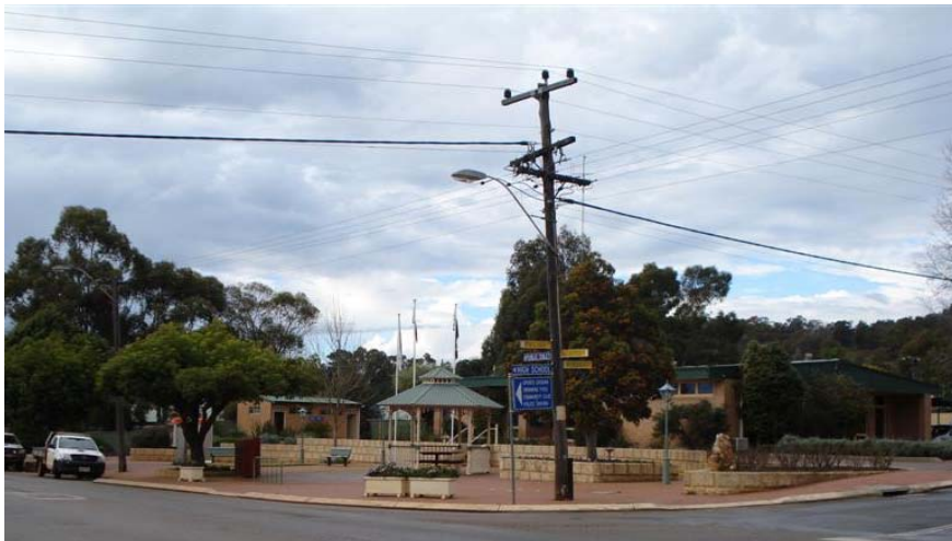
Photo 8: Overhead power lines
