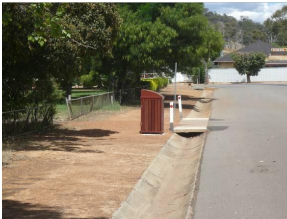
Current road side drainage infrastructure
