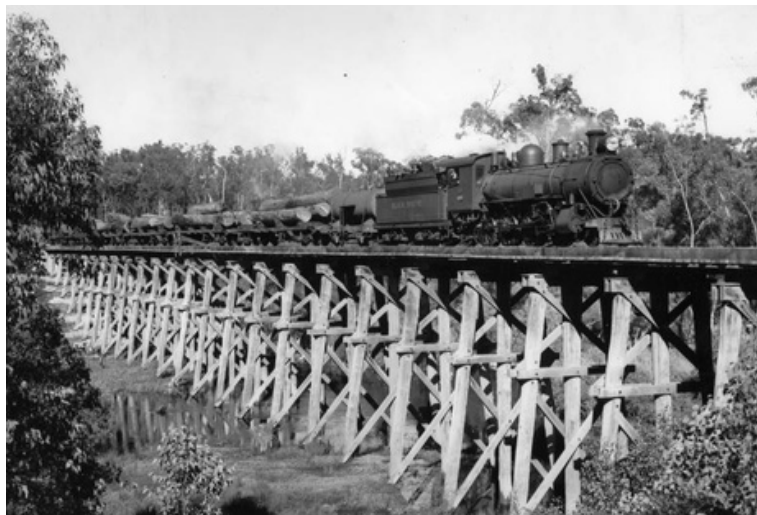
Image: Long Gully Bridge
