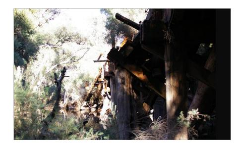
As a result of natural decay, the bridge has collapsed in the middle of the structure.
