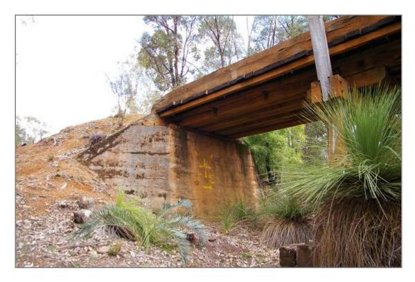
On the other side, concrete support has been installed. 28/06/10.
