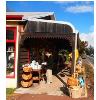
Verandah to shop front
