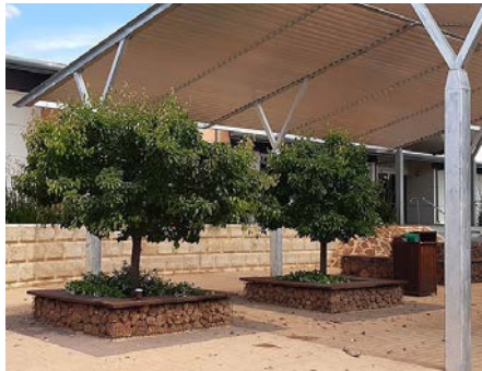
Existing materials & furniture reused in new plaza
